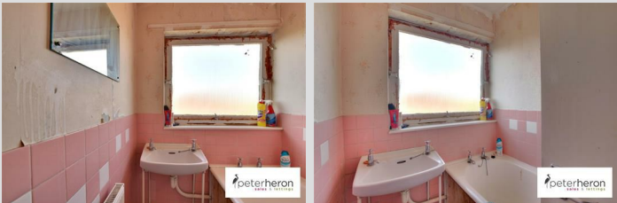
Wash hand basin, bath, radiator and a single glazed window.
